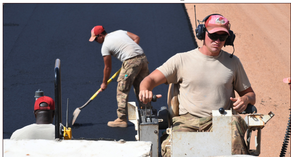
Staff Sgt. Channing Henry, 31st Expeditionary Rapid Engineer Deployable Heavy Operation Repair Squadron Engineer pavement and equipment journeyman, operates an asphalt paver on a test strip at Nigerien Air Base 201, Niger, Oct. 19, 2018. Airmen evaluate the equipment and materials several times before laying down the actual runway. (U.S. Air Force photo by Tech. Sgt. Rachelle Coleman)
