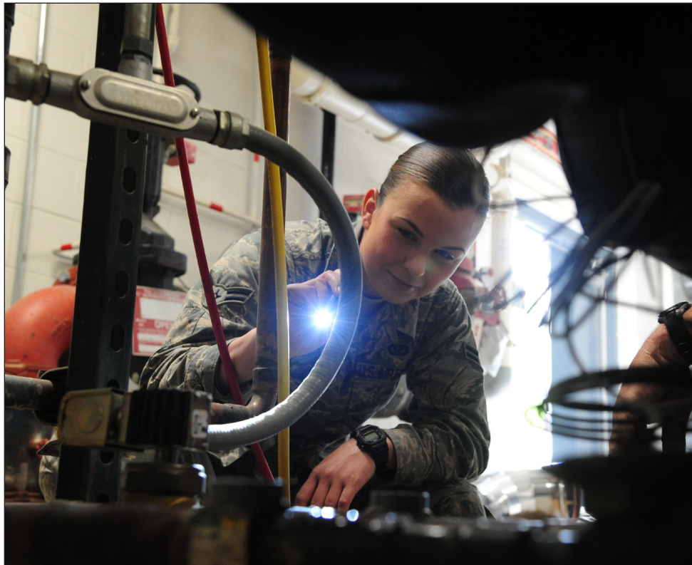
U.S. Air Force photo/Airman 1st Class Keenan Berry U.S. Air Force Airman 1st Class Dana Beck, a 509th Civil Engineer Squadron heating, ventilating and air conditioning apprentice, examines solder joints for leaks at Whiteman Air Force Base, Mo., April 20, 2016. Leaking solder joints could disrupt the air unit's cooling process and cause a system malfunction.
