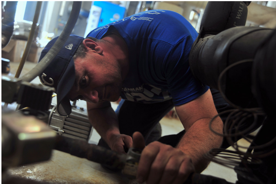
U.S. Air Force photo/Senior Airman Jovan Banks Tevin Gerke, a heating, ventilating, and air conditioning (HVAC) technician assigned to the 509th Civil Engineer Squadron, checks for coolant leaks after soldering replacement pipes at Whiteman Air Force Base, Mo., April 20, 2016. Depressurized pipes cause leaks which can lead to the loss of cooling capabilities in the air unit.
