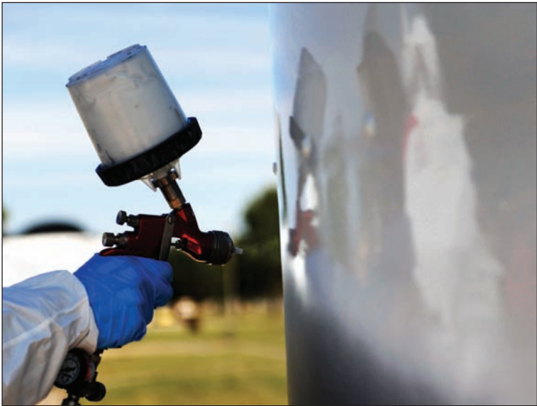
A low observable technician from the 509th Maintenance Squadron paints a Minuteman II Missile static display Sept. 14, 2015, at Whiteman Air Force Base, Mo. The missile was sanded, primed and painted in order to restore it.
