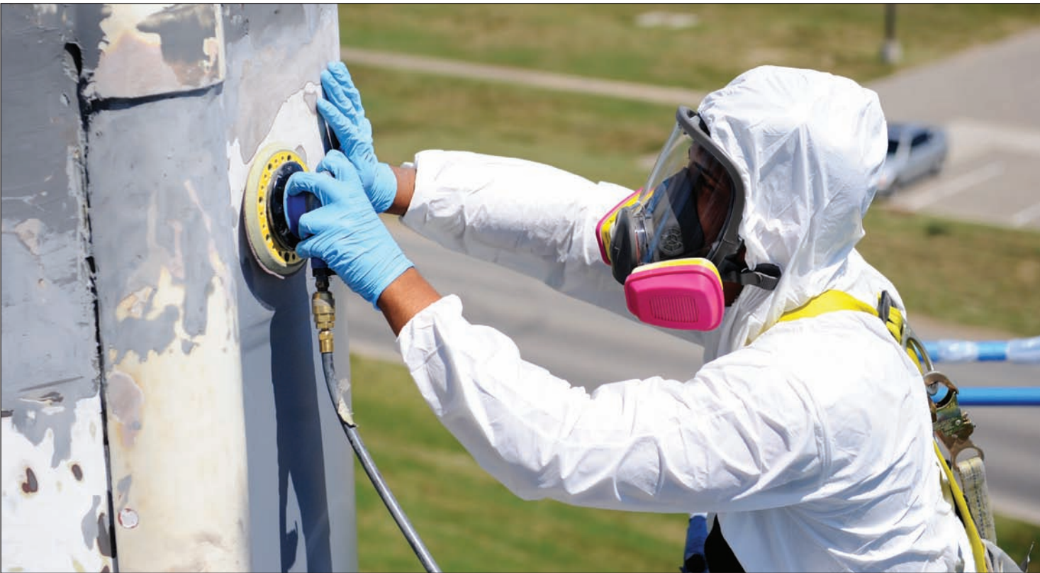
Senior Airman Carlos Colon, 509th Maintenance Squadron low observable technician, sands a Minuteman II Missile static display at Whiteman Air Force Base, Mo., Aug. 21, 2015. The missile was sanded, primed and then painted as part of the restoration process.
