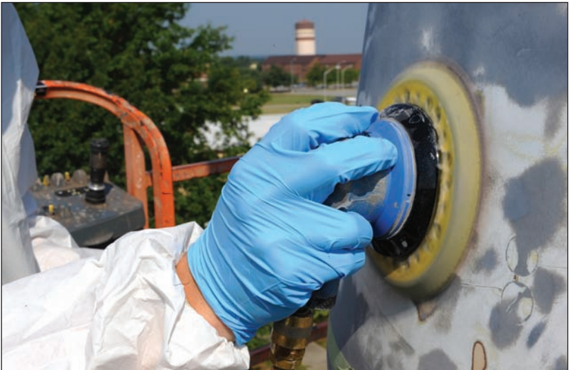
Senior Airman Carlos Colon, 509th Maintenance Squadron low observable technician, sands a Minuteman II Missile static display at Whiteman Air Force Base, Mo., Sept. 1, 2015. As part of the restoration process, the missile was sanded, primed and painted.
