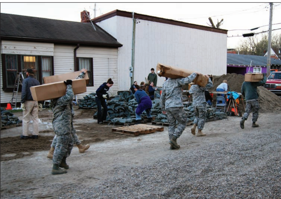
Members from the Missouri Air National Guard hoist rolls of plastic sheeting for use on a sandbag levee in Clarksville, Mo., April 19, 2013, as part of the Guard response to flooding along the Mississippi River. About 50 Guardsmen from St. Louis were mobilized to help construct the levee, which spans about 1,500 feet.
