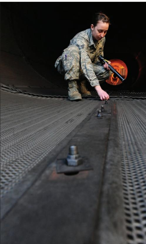
Senior Airman Kaitlyn Fawber, 509th Maintenance Squadron aerospace propulsion journeyman, inspects a test cell rivet, Feb. 13. The test cell is a \$2.9-million-facility used by jet engine mechanics to test the serviceability of jet engines.
