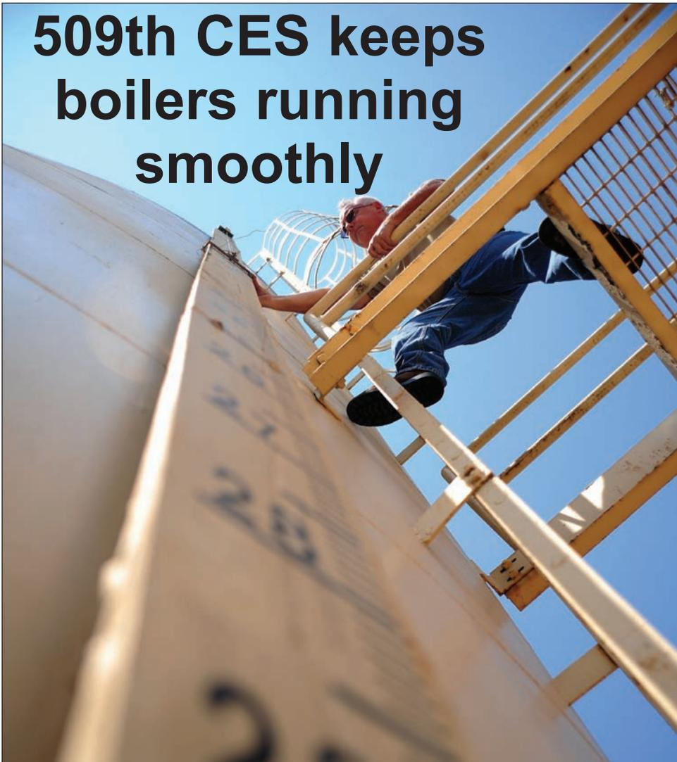
Paul Ross, 509th Civil Engineer Squadron central heat plant project manager, checks the level of liquid in a 100,000 gallon diesel fuel tank, Aug. 27. This is one of three fuel tanks used as an emergency back-up to support the boilers that provides heat on base.
