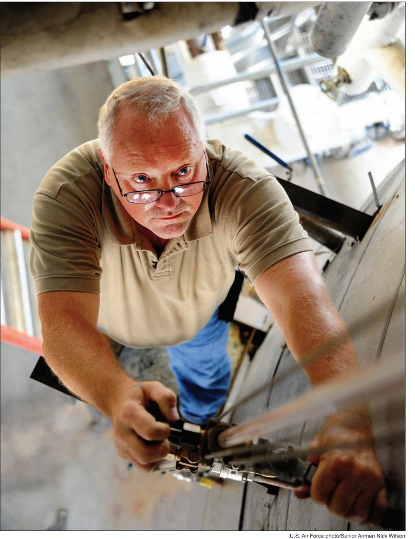
Paul Ross, 509th Civil Engineer Squadron central heat plant project manager, inspects sight glasses on a condensate receiver tank, Aug. 27. The purpose of the inspection is to ensure the receiver tank is mission capable for continual use. See page 3 for more photos.
