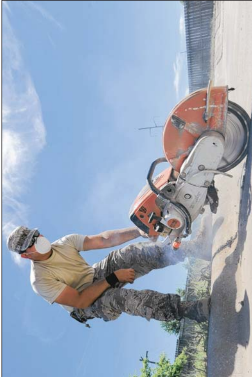
Senior Airman Travis Knighten, 509th Civil Engineer Squadron pavement and equipment operator, grinds out tar sealant from the crevices of a parking lot. Tuesday. Repairing the sealant protects the concrete from weather and helps prevent cracking.
