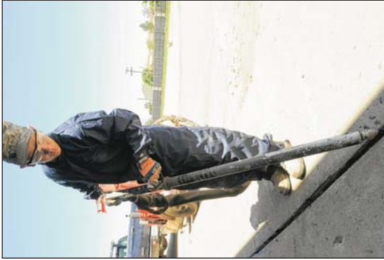
Senior Airman Travis Knighten, 509th Civil Engineer Squadron pavement and equipment operator, grinds out tar sealant from the crevices of a parking lot. Tuesday. Repairing the sealant protects the concrete from weather and helps prevent cracking.
