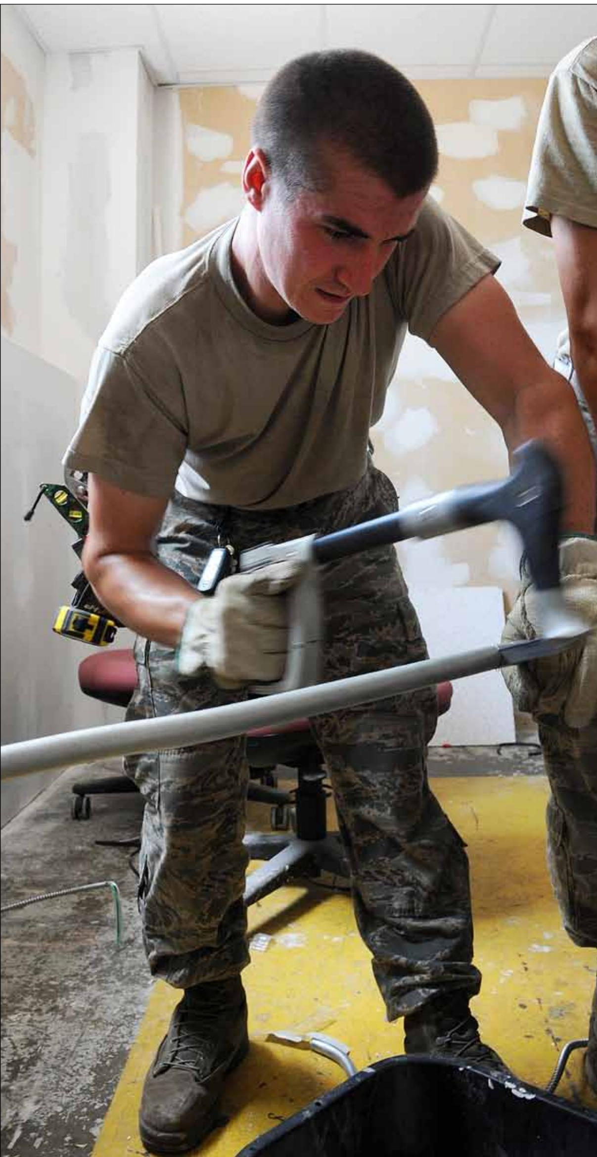
U.S. Air Force Senior Airman Eric Miller, a 509th Civil Engineer Squadron electrical systems journeyman, saws a conduit for new wiring at Whiteman Air Force Base, Mo., July 5, 2016. Metal conduits are a wiring method that provides mechanical protection to the enclosed electrical system.
