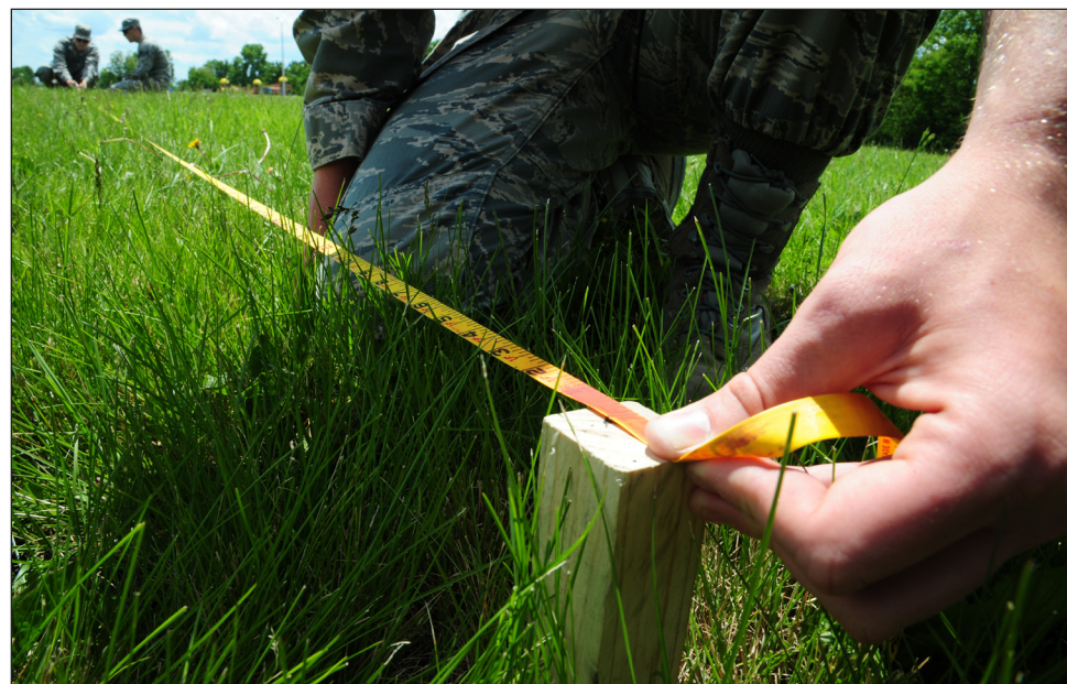
Members with the 509th Civil Engineer Squadron geobase shop measure the length of a building's foundation at Whiteman Air Force Base, Mo., May 18, 2016. Engineering technicians must obtain accurate measurements from each building's corner to plot the next coordinate for the building foundation.
