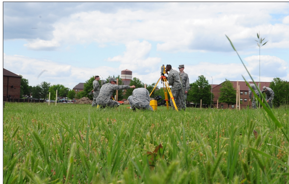
Engineering technicians from the 509th Civil Engineer Squadron (CES) geobase shop establish a building foundation at Whiteman Air Force Base, Mo., May 18, 2016. In a contingency environment, the geobase shop is responsible for assembling the foundation before CES heavy equipment operators lay concrete pads.
