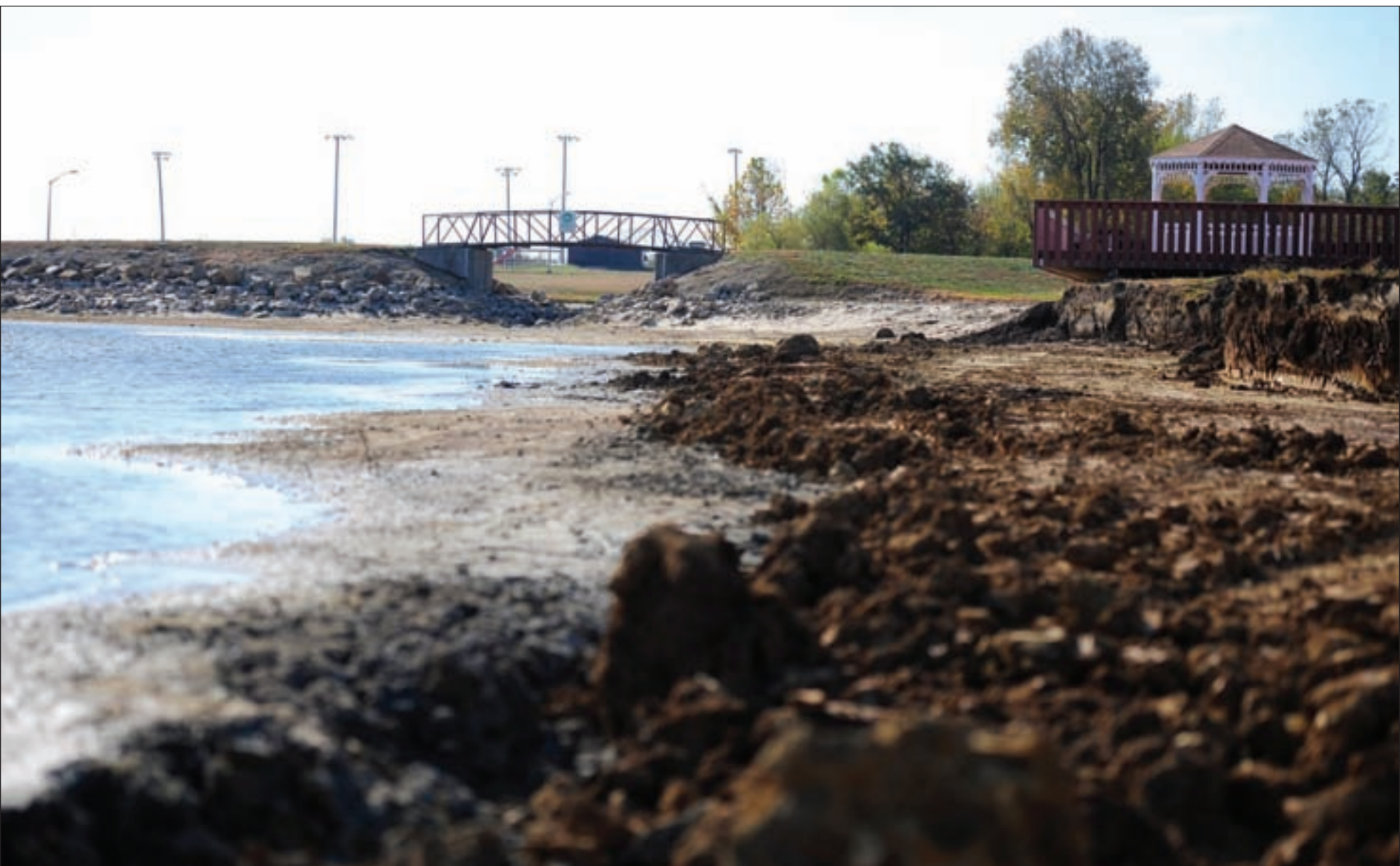
The shoreline at Ike Skelton Lake is exposed Oct. 20, 2015, following a draining performed by contractors at Whiteman Air Force Base, Mo. The water level was lowered as part of an on-going project which includes the installation of a brick wall along the water's edge. Following the shoreline reinforcement, the water level will be raised higher than normal, which decreases the algae and weed growth in the shallow areas of the pond. The shoreline is scheduled to be closed until December 2015.
