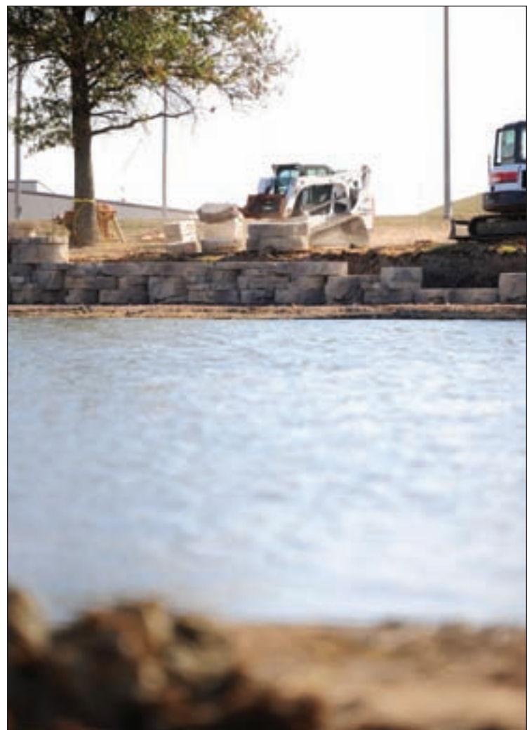
A contractor operates a Bobcat skid-steer loader to transfer bricks near the edge of Ike Skelton Lake Oct. 20, 2015, at Whiteman Air Force Base, Mo. To decrease algae and weed growth in shallow areas of the pond, the shoreline is being reinforced with a brick wall and is scheduled to be closed until December 2015.
