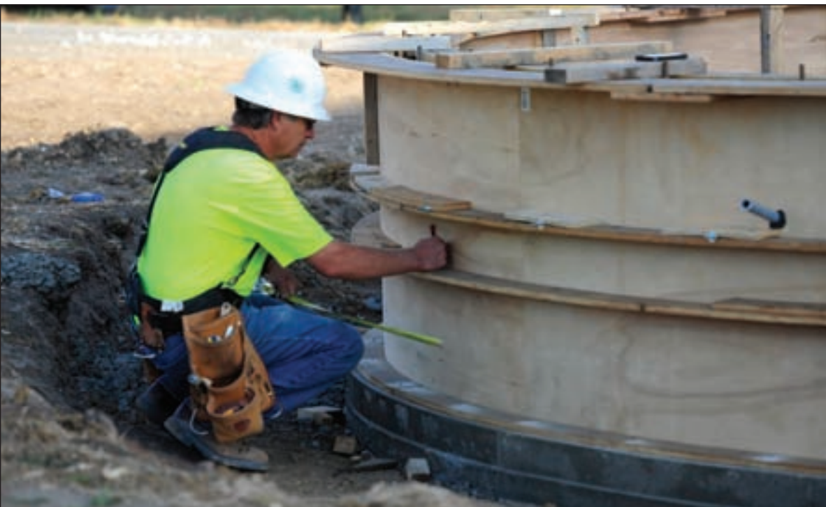
George Arney, a construction carpenter, marks drill holes in a new fire pit located near the Ike Skelton pavilion Oct. 21, 2015, at Whiteman Air Force Base, Mo. Form ties are inserted into the holes and used to prevent the structure from spreading when concrete is poured into the seating and supporting wall. The pavilion and stage area is scheduled to be closed until mid-December 2015.
