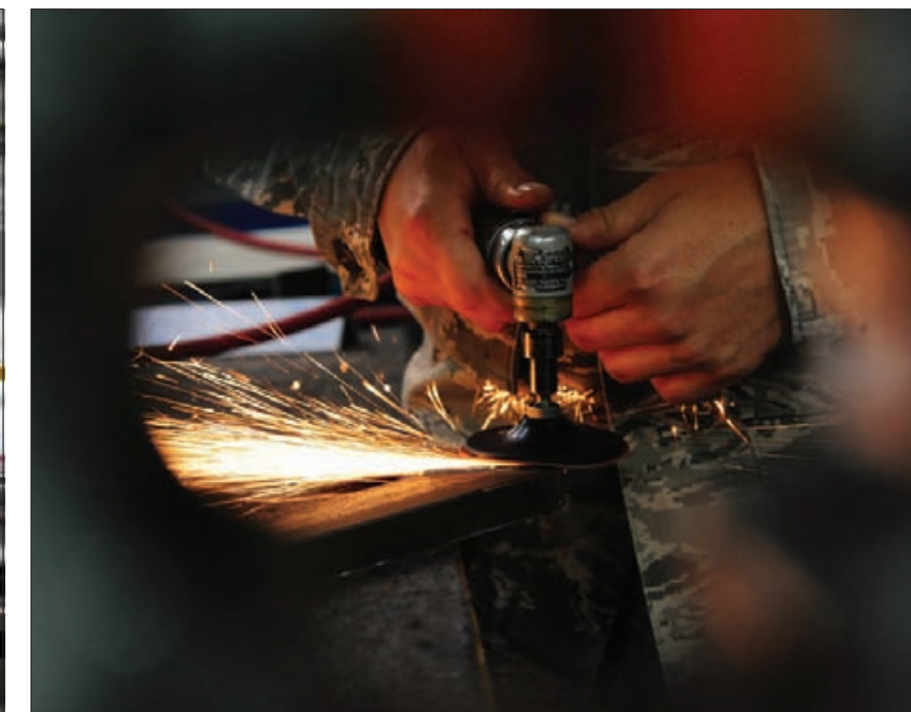
U.S. Air Force A.J. Long, 495th Fighter Group structural maintenance technician, grinds a door frame at Whiteman Air Force Base, Mo., Sept. 15, 2015. This process is done to clean up weld marks from the procedure.
