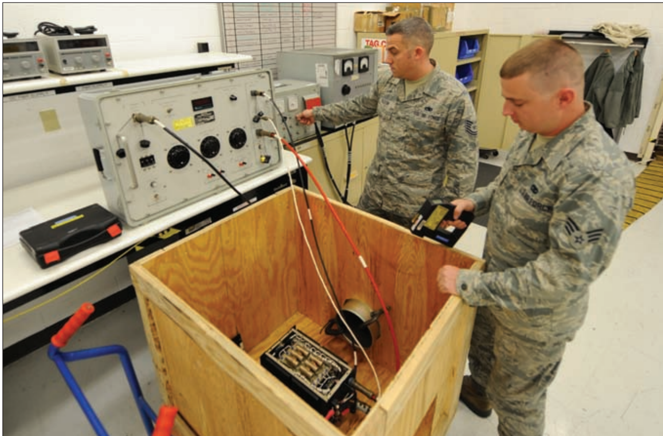
Tech Sgt. Shawn Bloom and Senior Airman Colby Nash, 509th Maintenance Squadron electrical and environmental systems specialists, perform a check on a transformer rectifier to ensure it is working properly before placing it back into supply at Whiteman Air Force Base, Mo., Nov. 25, 2014. Members of the shop also assist fuels, engines, hydraulics and the crew chiefs with various troubleshooting and repairs.
