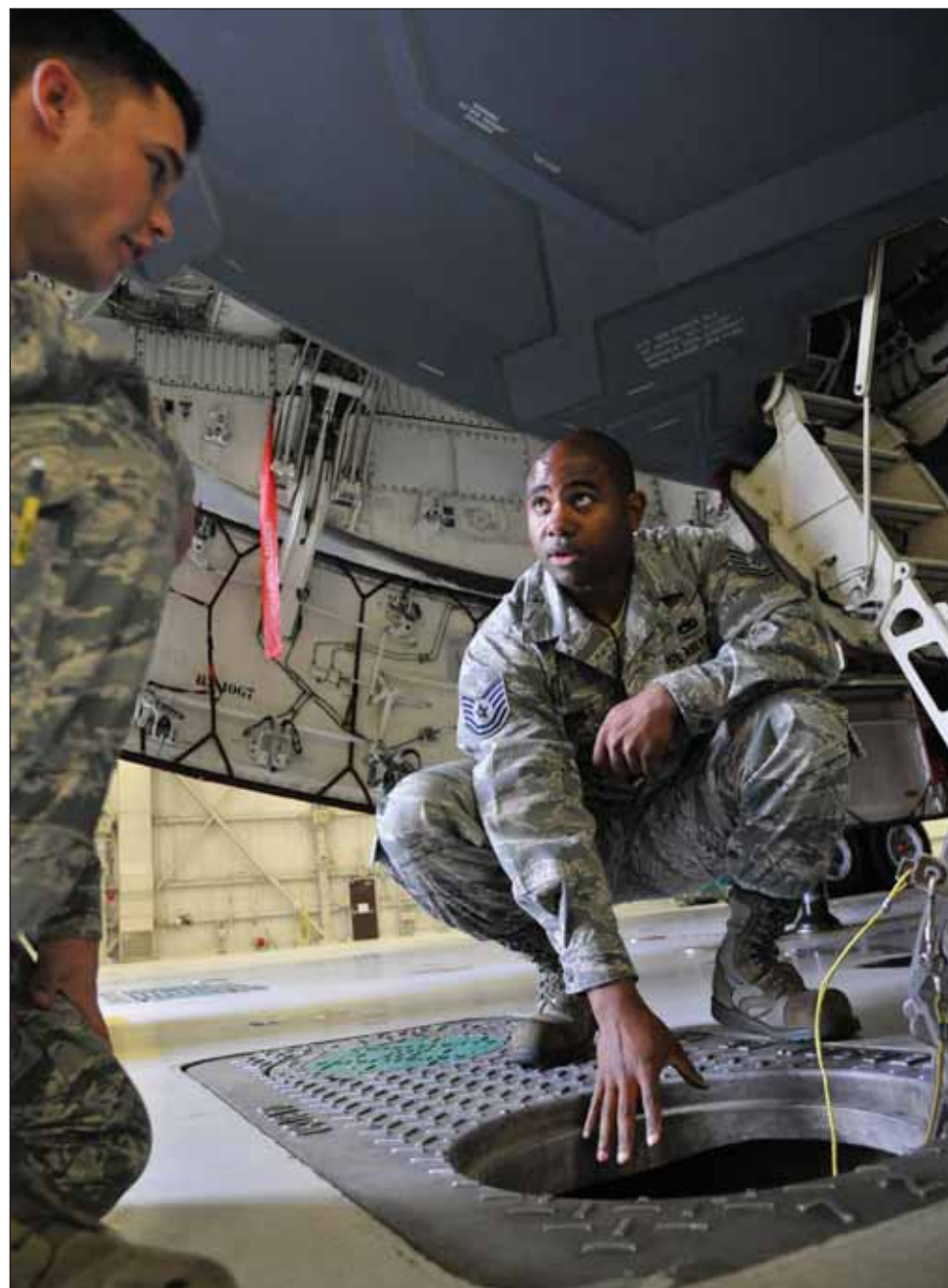
U.S. Air Force Tech. Sgt. Broderick Jones, 509th Aircraft Maintenance Squadron aircraft electrical and environmental systems craftsman, explains each dock’s ability to provide cooling to Airman 1st Class Evan Miesner, 509th AMXS electrical environmental apprentice, at Whiteman Air Force Base, Mo., June 10, 2014. Each dock is capable of providing cooling to the aircraft for operational checks and maintenance.
