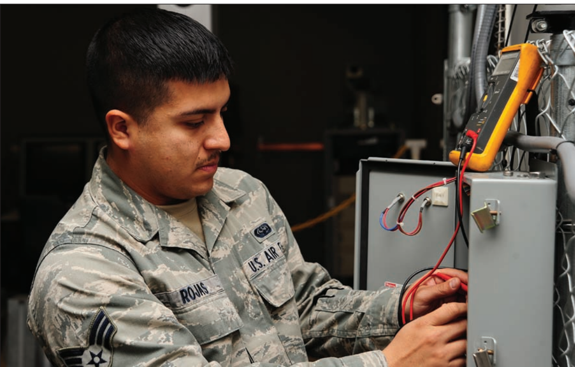
Senior Airman Luis Rojas, 509th Communications Squadron intrusion detection systems technician, checks electrical resistance with a multimeter to ensure an alarm is secure. If the electrical current on the alarm is not at the correct measurement, then the device will not function properly.
