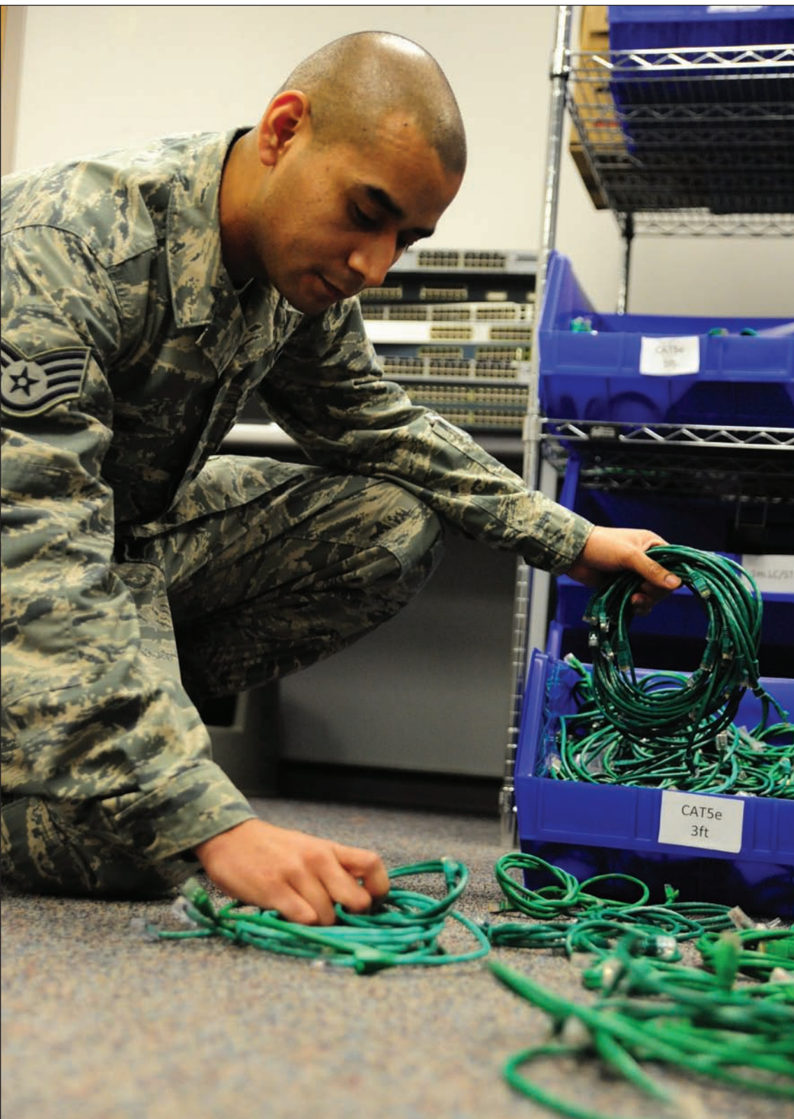
Staff Sgt. Gabriel Lopez, 509th Communications Squadron network technician, accesses cables to activate ports for a customer at Whiteman Air Force Base. Network technicians are responsible for maintaining all types of networks on base and allowing Airmen to access the Global Information Grid.
