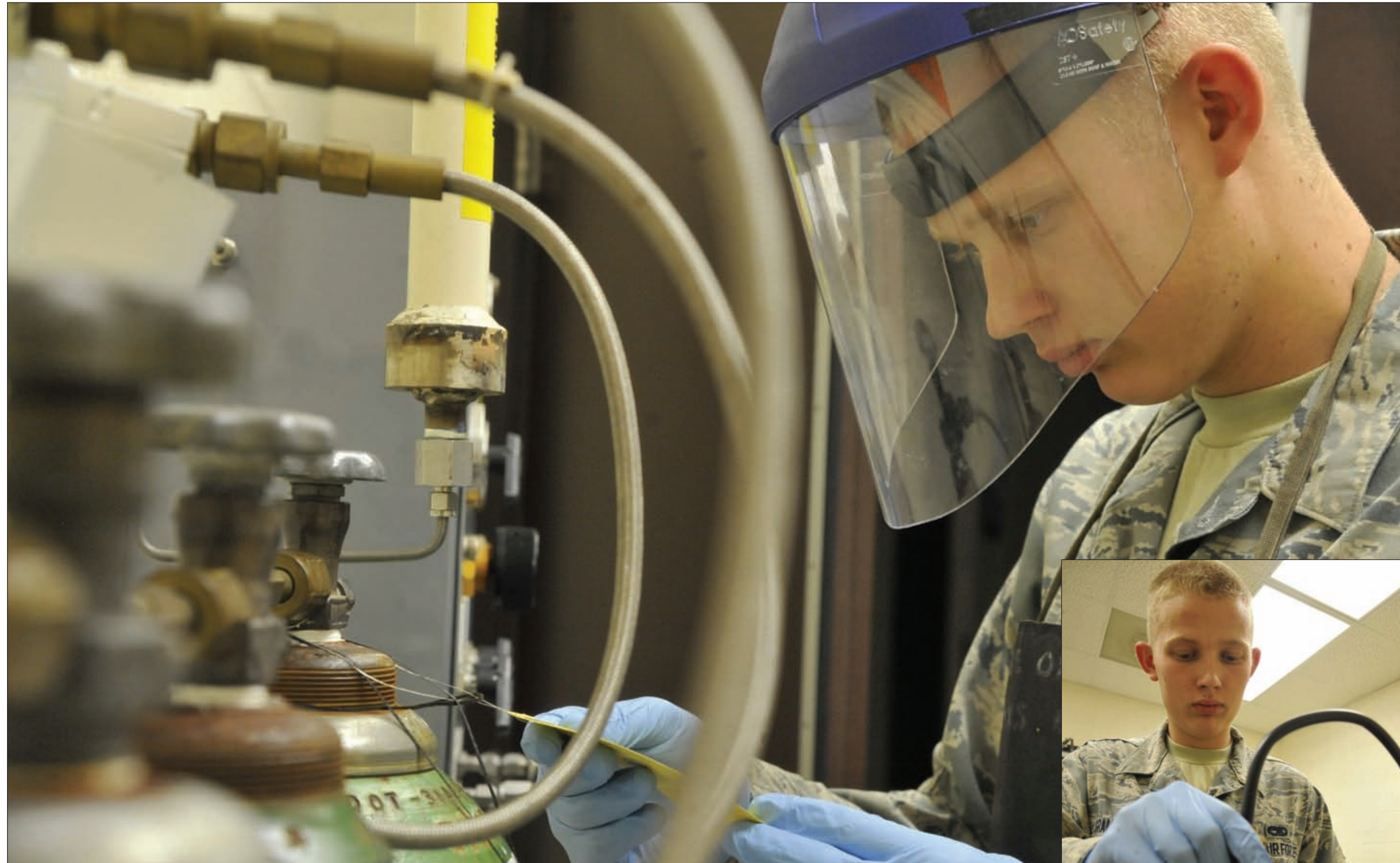
U.S. Air Force Airman 1st Class Chad Grauerholz, 509th Maintenance Squadron electrical environment technician, inspects an oxygen servicing station at Whiteman Air Force Base, Mo., Oct. 15, 2013. This process is designed to ensure the oxygen has not expired and there is enough pressure to fill up emergency oxygen cylinders.
