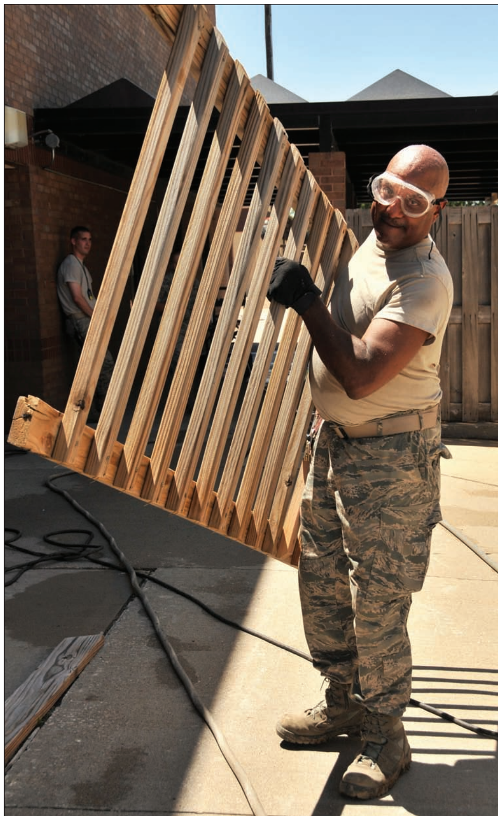
Master Sgt. Jonathan Allen, a plumber with the 131st Civil Engineer Squadron, prepares a leased trailer to be returned to its owner June 26, 2013, at Whiteman Air Force Base, Mo. With a background in carpentry, Allen's knowledge of how things are put together was helpful in completing the project.
