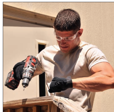
Staff Sgt. Alex Zeman, a heating, ventilation and air conditioning journeyman with the 131st Civil Engineer Squadron, removes screws from the back deck of a leased trailer June 26, 2013, at Whiteman Air Force Base, Mo. Zeman and two other Airmen from his squadron traveled here from Lambert Air Guard Station near St. Louis to team up with the 509th CES and get the trailer back to its owner.
