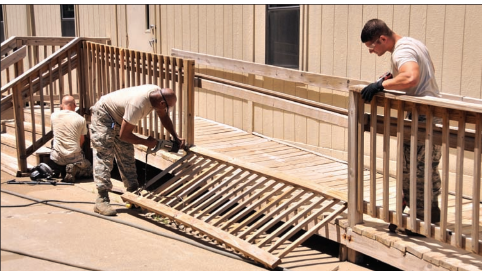
From left to right: Senior Airman Royce Koch, Master Sgt. Jonathan Allen and Staff Sgt. Alex Zeman, from the 131st Civil Engineer Squadron, disassemble the back porch of a leased trailer June 26, 2013, at Whiteman Air Force Base, Mo. This was the first time the 131st teamed up with the 509th Civil Engineer Squadron on a joint project of this scale.
