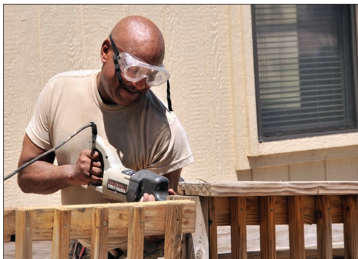
Master Sgt. Jonathan Allen, a plumber with the 131st Civil Engineer Squadron, starts taking apart the back deck of a leased trailer June 26, 2013, at Whiteman Air Force Base, Mo. The 131st, based out of Lambert Air Guard Station near St. Louis, collaborated with their active-duty counterparts from the 509th CES at Whiteman on this project.
