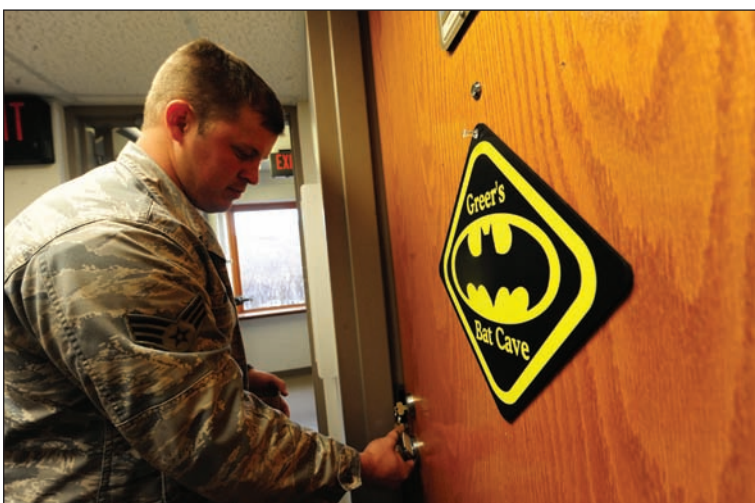
Senior Airman David Bandy, 509th Civil Engineer Squadron structures journeyman, re-keys a broken lock on a dorm room door, March 6. Bandy and other locksmiths on base are responsible for ensuring all base facilities are both secure and accessible.
