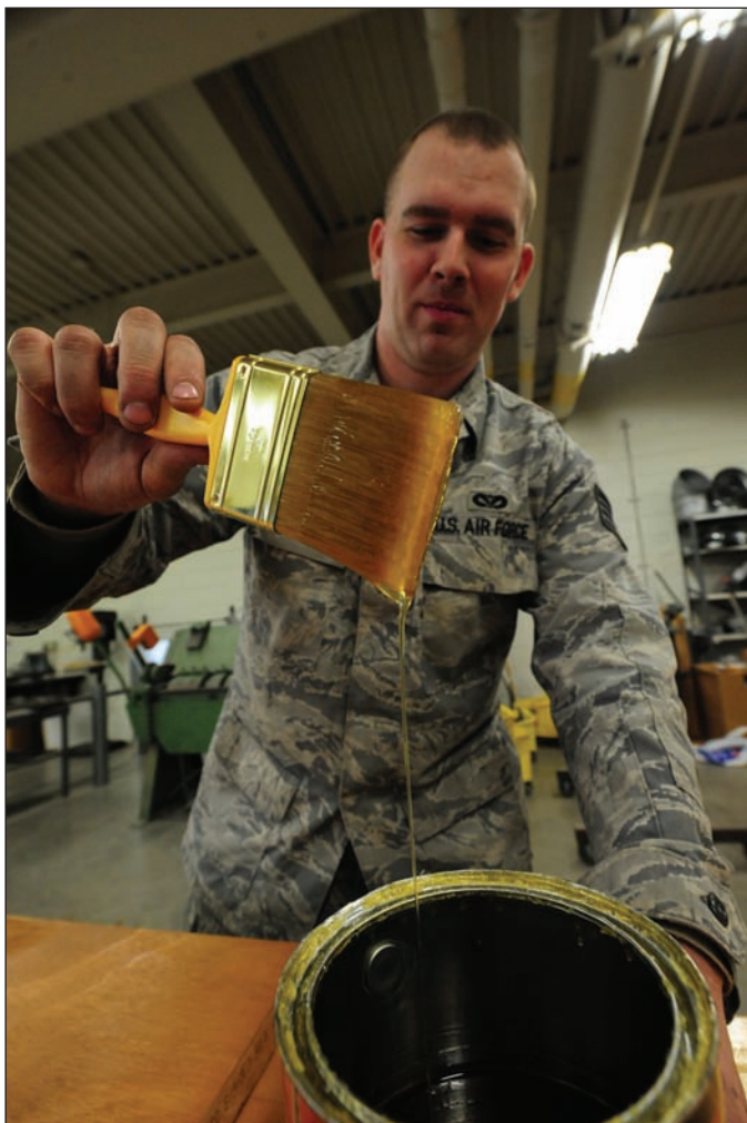
Staff Sgt. Adam Boyd, 509th Civil Engineer Squadron structural supervisor, dips a brush in polyurethane before polishing a wooden door, Feb. 27. The polyurethane prevents moisture from absorbing into the wood.
