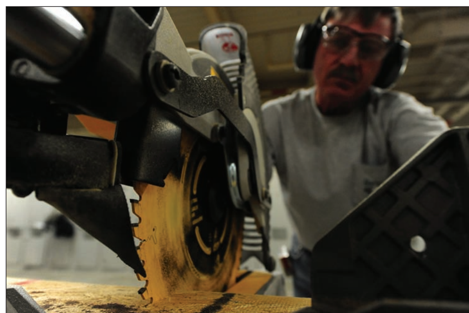
Albert Cote, 509th Civil Engineer Squadron carpenter, uses a compound miter saw to cut a piece of wood for a door frame, Feb. 27. The door frame will be used to repair a temporary lodging facility.
