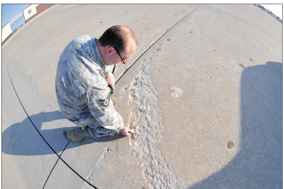
Staff Sgt. Timothy Cole, 509th Operation Support Squadron Airfield Management operation supervisor, inspects a spall, Feb. 6. A spall is a defect in the concrete surface caused by erosion or strong vehicle use; as it starts to deteriorate, the concrete starts to break into small pieces, creating FOD.
