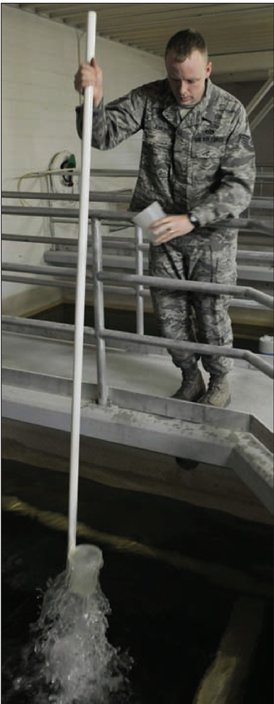
Tech. Sgt. Jason Jenkins, 509th Civil Engineer Squadron water fuels systems supervisor, draws a sample of water from one of the four sand/anthracite filters that are capable of filtering 1,800 gallons per minute at the water treatment plant. Even though ground water is typically safer than surface water, filtration is the only method known to remove pathogens in the treatment process.
