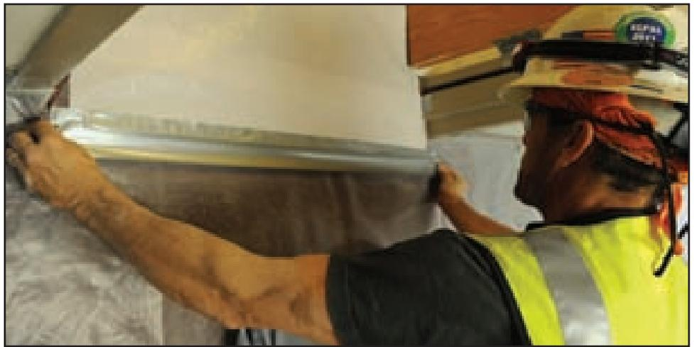
A contractor from Far East Contracting uses duct tape to tape plastic down to the floor in Atlantis Hall Jan. 10. Plastic covering the floor allows easy clean up for contractors. Atlantis Hall is part of a \$7.8 million renovation project to include upgraded heating and air conditioning systems, plumbing and installation of new fire safety sprinklers.
