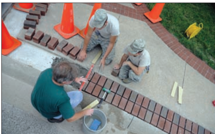
Senior Airman Isaac Fifer, Airman 1st Class Aaron Avila and Mr. Dennis Spear, 509th Civil Engineer Squadron structure shop technicians, work together to level a brick pathway in front of the 509th Bomb Wing building here July 6. Mr. Spear was teaching the Airmen techniques to ensure quality brick work and a lasting product.
