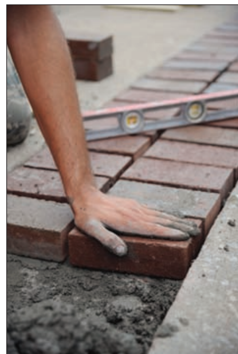
Senior Airman Isaac Fifer, 509th Civil Engineer Squadron structure shop technician, lays a brick while completing a new pathway in front of the 509th Bomb Wing building here July 6. Throughout the Midwest seasons, water trapped in between the bricks caused erosion and the surface becomes uneven.
