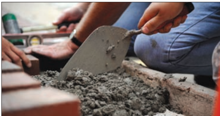
An Airman from the 509th Civil Engineer Squadron structure shop spreads mortar to lay brick in front of the 509th Bomb Wing Building here July 6. An even spread of mortar is important when laying brick, ensuring a smooth pathway and level surface.
