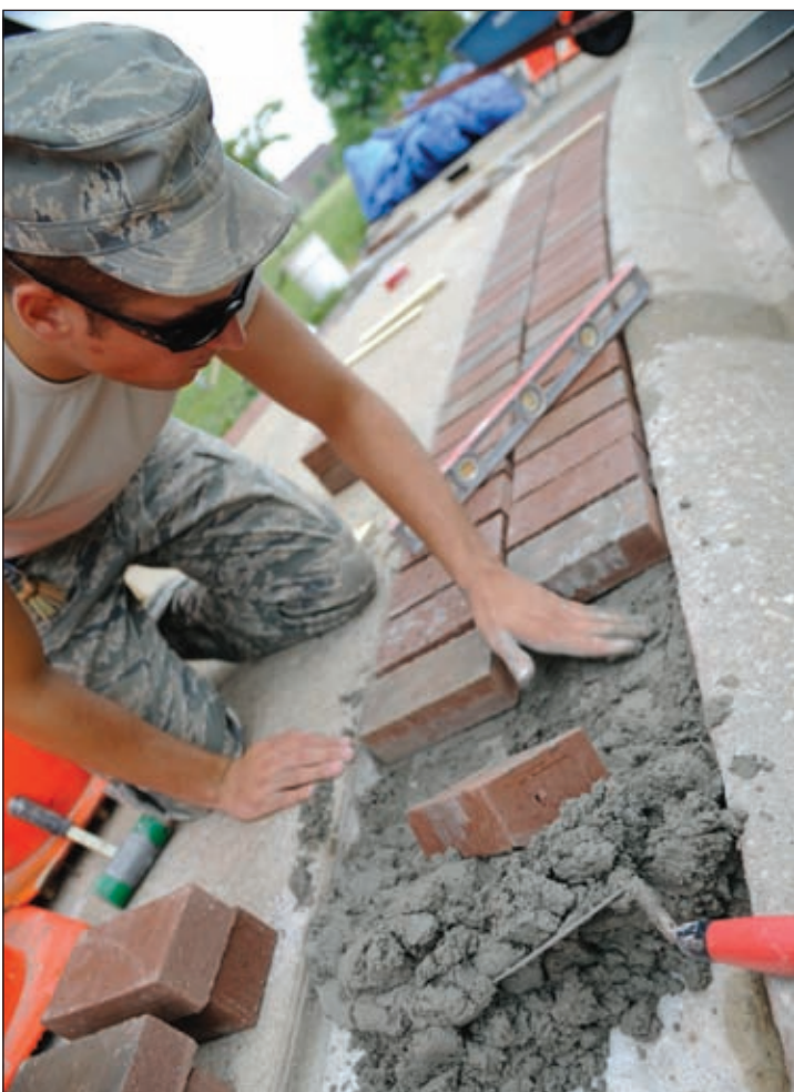
Senior Airman Isaac Fifer, 509th Civil Engineer Squadron structure shop technician, packs mortar in an empty slot before placing a brick on the new pathway here July 6. Mortar is essential in brick laying, binding bricks together and drying into a sturdy structure. It is typically made from a mixture of sand, cement and water.
