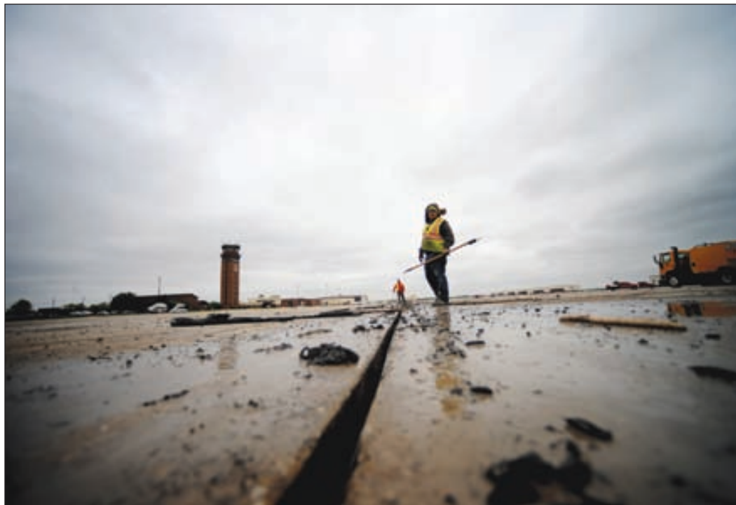
Far left: Bell Contracting Inc. employees discuss construction operations on the Whiteman flightline April 26. Left: A Bell Contracting Inc. employee looks across the Whiteman flightline as him and his co-workers make progress resealing the grooves between the concrete slabs that make up Whiteman's flightline April 26. Below: A Bell Contracting Inc. employee operates a high powered circular saw to ensure the last bits of old silicone and foam have been removed from the grooves in between the concrete slabs that make up Whiteman's flightline before resealing them April 26.
