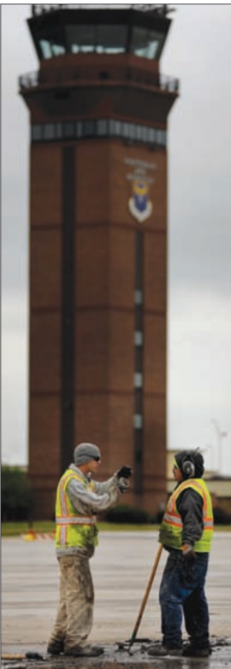
Above: A Bell Contracting Inc. employee tightens his grip as he scrapes between grooves of the concrete slabs that make up Whiteman's flightline ensuring any old silicon and foam has been removed before placing new silicone and foam April 26. Right: A Bell Contracting Inc. employee endures dirt and grime being blasted into his face as he sprays a pressure washer in the grooves of the concrete slabs that make up Whiteman's flightline ensuring any old silicon and foam has been removed before placing new silicone and foam April 26. BCI contractors are repairing large portions of Whiteman's flightline over the next several weeks in order to keep it in operational condition for flight operations.
