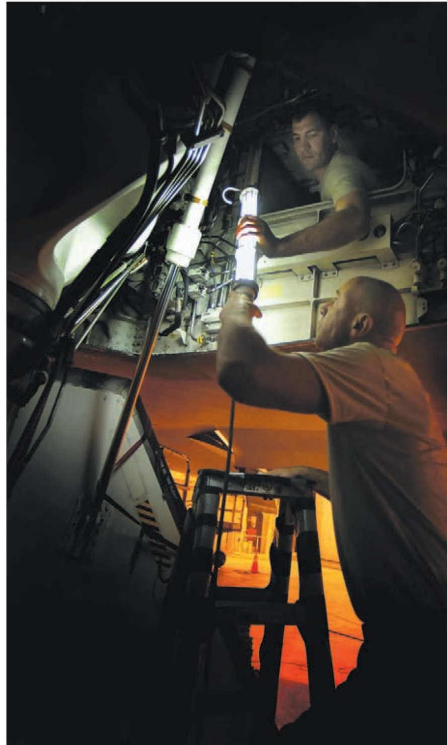
U.S. Air Force photo by Senior Airman Kenny Holston Master Sgt. Andrew Hensley, 131st Maintenance Squadron NCO in charge fuels system repair shop hands a fluorescent light to Senior Airman Joseph Mango, 509th Maintenance Squadron fuels system technician as he prepares to crawl into the blow out bay of a B-2 Spirit to perform an inspection April 26. Inspections such as these ensure the integrity of the fuel system keeping the aircraft combat ready.
