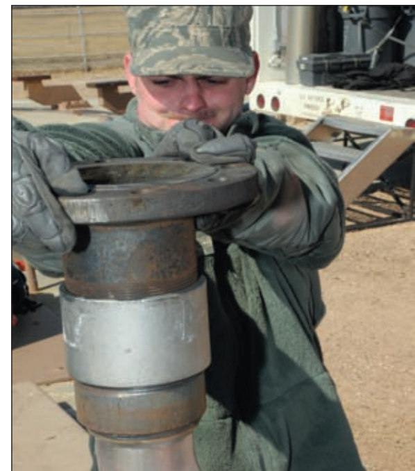
U.S. Air Force photo by Blaze Lipowski F. E. WARREN AIR FORCE BASE, Wyo. -- Senior Airman David Reynolds, 90th Maintenance Squadron, installs the exhaust shroud on the new diesel engine before lowering it into position as the launch facilities back-up power supply March 18.
