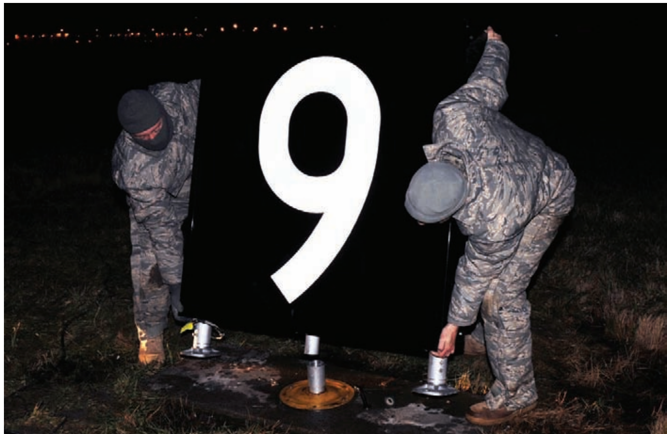
Airman 1st Class Raymond Reidenbach and Airman 1st Class Corey Logsdon, 509th Civil Engineer Squadron electrician, are setting the new light-emitting diode distance-remaining marker in place next to the runway. The LED fixtures are designed to cut energy costs by 70 percent.
