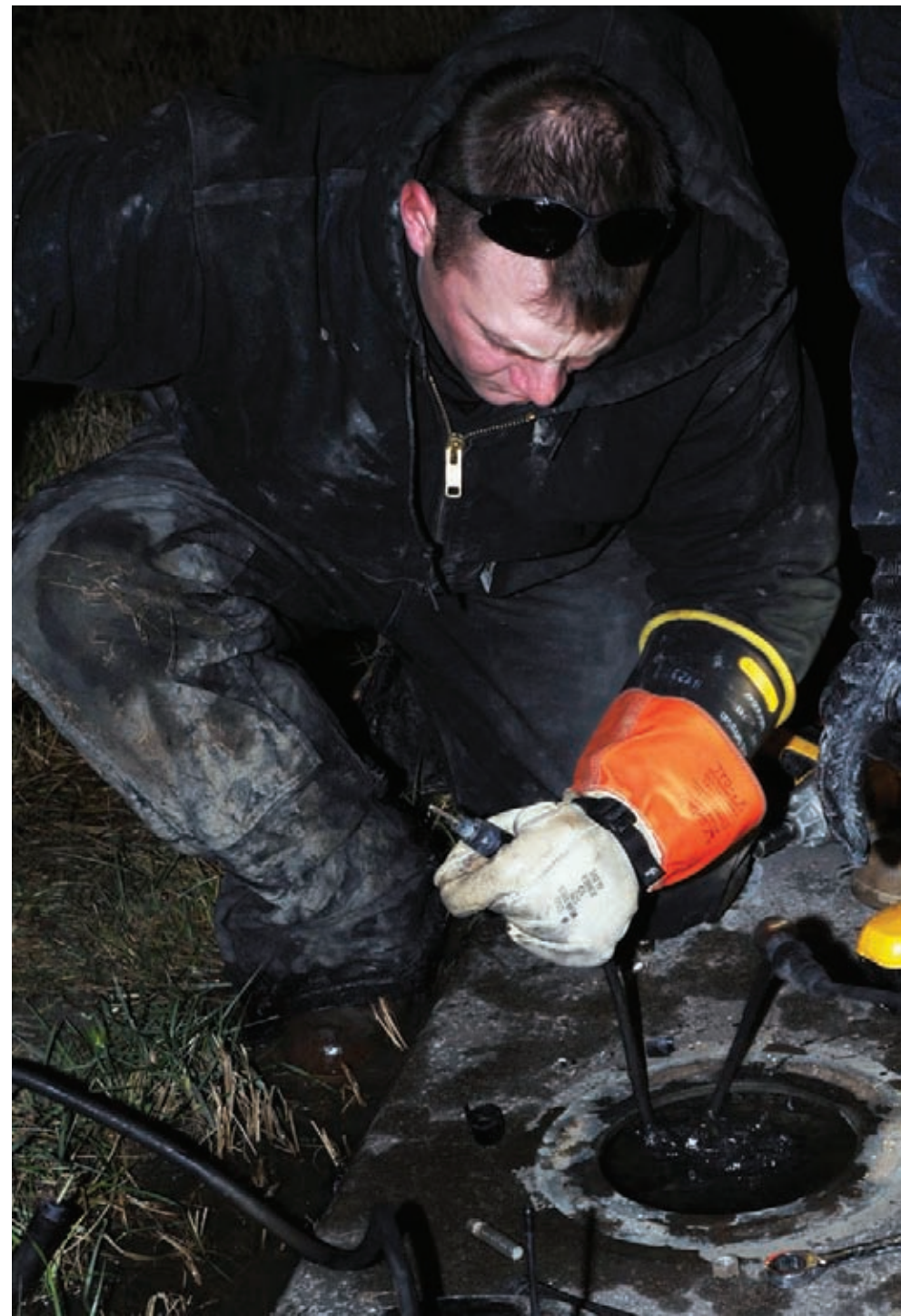
Staff Sgt. James Thompson, 509th Civil Engineer Squadron electrician, connects new transformer to circuit for runway-distance-remaining marker on 30 Nov.
