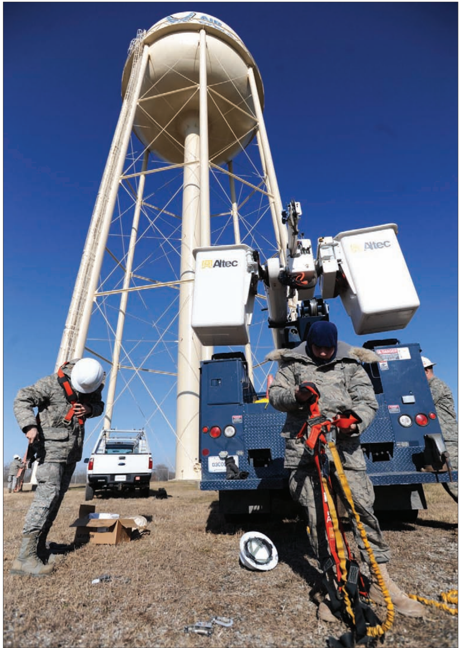
Airman 1st Class Francisco Villa and Corey Logsdon, 509th Civil Engineer Squadron electric technicians, put on safety harnesses, hard hats and cold weather gear to climb the 215-foot water tower behind them, Dec. 1. Airman Villa and Airman Logsdon serviced the rotating beacon and tower lights for flight safety here.
