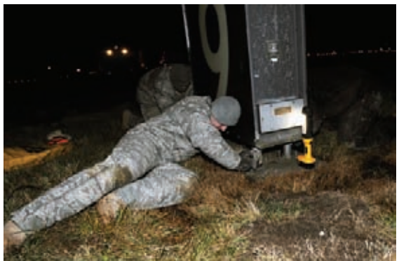
Airman 1st Class Corey Logsdon, 509th Civil Engineer Squadron electrician, prepare to remove an old runway-distance-remaining marker by loosening anchor bolts and upgrade it to a new light-emitting diode fixture. The LED fixtures are designed to cut energy costs by 70 percent.
